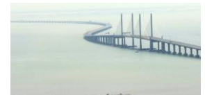
Penang Second Bridge (around RM4.5bn)
